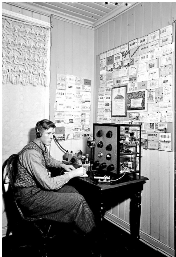
Photographs taken of Gunnar Eriksen, LA6K (left) and Erling Hoel, LA6B (right) at the operating position of their pre-war amateur radio station. Both transmitters (on the table right) shares its construction with the 'Tynset 1940 campaign transmitter' in this chapter and is believed to be an example of a design published in a radio amateur magazine.
