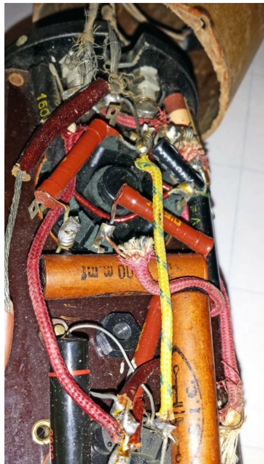
Close up view of bottom showing the fragile and brittle state of the original wiring. (right)
