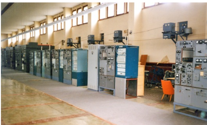
Inside view of the transmitter hall of the MFS HV A transmitting site located in Zeesen near Berlin. (Left) Transmitters with a power ranging from 1 to 20 kW were in use. These were of Russian and GDR manufacture. The main HV A receiving site was in Wernsdorf. Both sites were also used for passing traffic for the Short Wave Communication System 32210.
