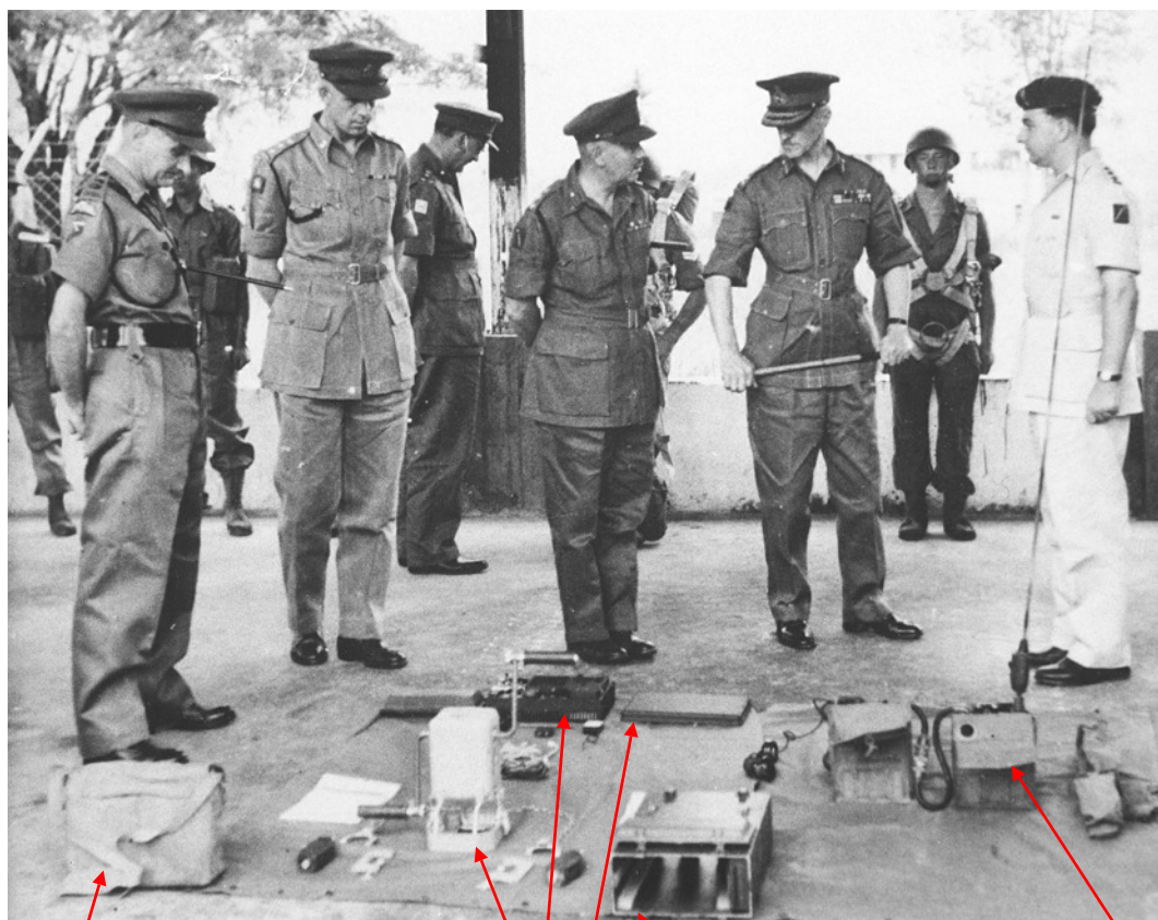
Mk. 810A hand/pedal generator Canvas bag for Mk. 810A Mk. 122 Mk. 122 top cover Immersion proof container Mk.122 Wireless Station A 510
