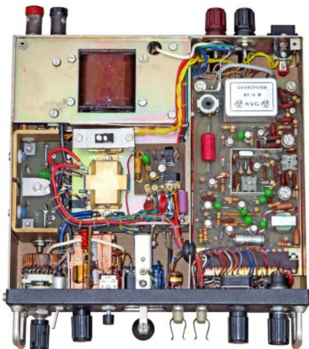
Bottom view of the set (left) showing second receiver board with 9MHz IF crystal filter, detector, BFO and AF stages. Note the use of a W-German KVG type XF9-B crystal filter. A Haller transmit-receive relay was fitted centre left just below the mains transformer, padded in foam plastic.
