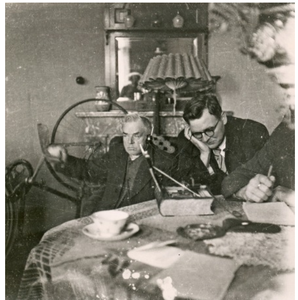
Listening to an Allied broadcast station with a clandestine radio hidden in a book. Note that the listener at the left is operating the crank of an upturned bicycle to power the receiver from a dynamo.
